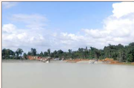
CNPC's Reservoir at Made Island.
