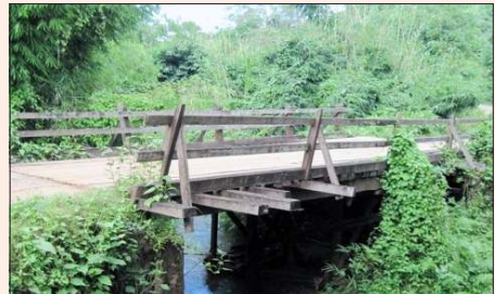
Belly Bridge on the road from Myitkyina to Myitstone before
