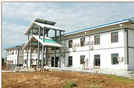
Hospital under construction by CNICO.
